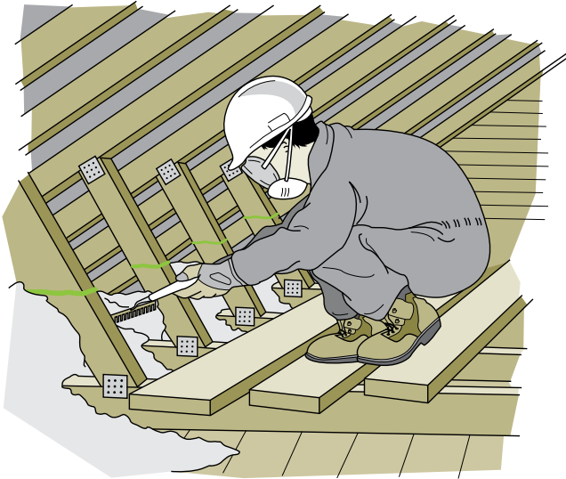
Figure 5-14 Installing loose-fill insulation
